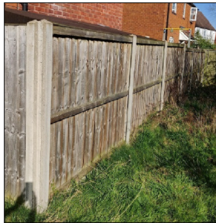
1.8m high concrete post and timber fence
